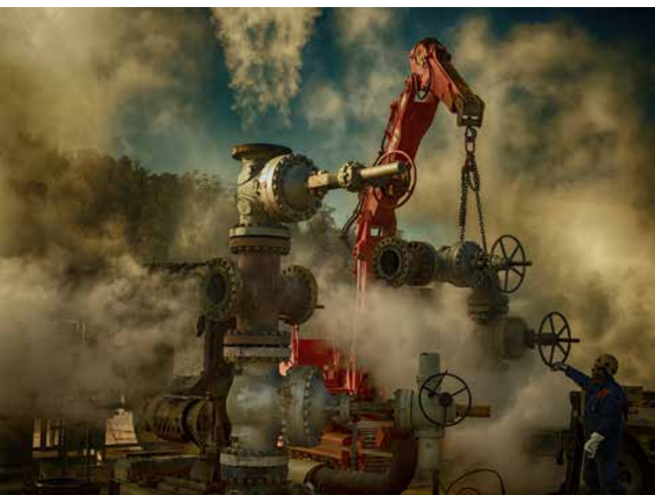
Sartori Fabio Geothermal works 2021
